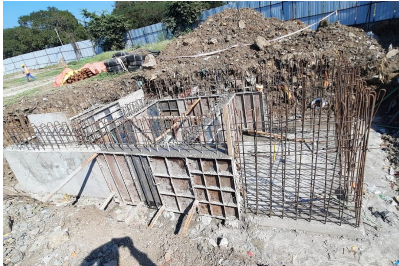
AFCONS INFRASTRUCTURE LTD., Mumbai metro line 05, Kapurbawdi to Dhamnkar naka, Casting yard civil work, Sedimentation tank and Pipe culvert work
